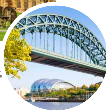
Tyne Bridge, Newcastle
