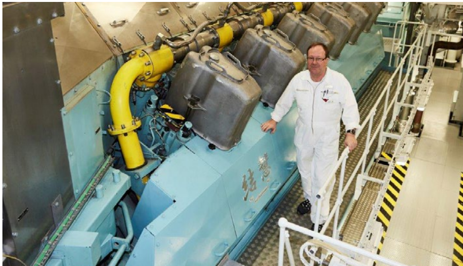
The dual-fuel engine on AIDAprima. LNG flows through the yellow pipes to the cylinders.
